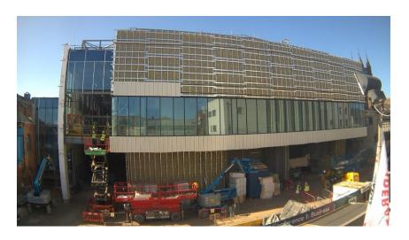
External cladding is now nearing completion with the main elements left to finish in this regard being the remainder of the Terracotta cladding to the front elevation of the building, due to be complete mid-June 2021.
